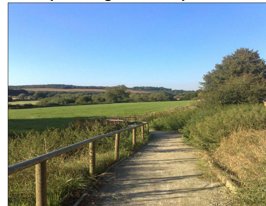
Examples of gravel footpath construction
