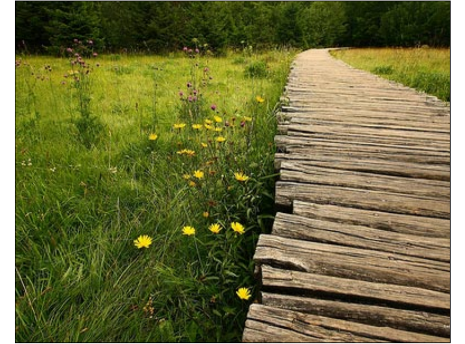
Examples of boardwalk construction
